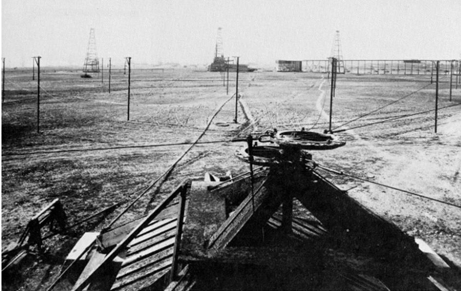
**Figure 4** At the Company Site, Photo Showing Jack Lines Supported by Wood and Metal Jack Line Swings, Looking Towards the Jack Plant, 1974
